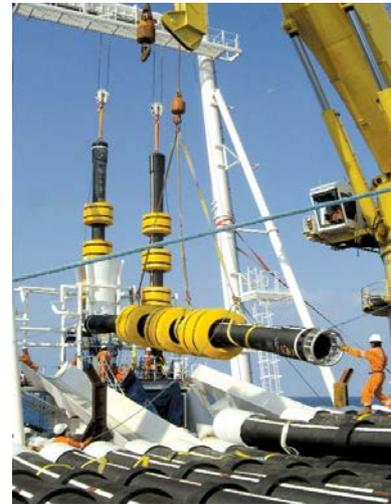
The hose deployment system was tested at Caley's quayside facility before being shipped for integration onboard the SBM Normand Installer. The system was successfully used to deploy two offloading lines without disruption to the assembly process.
